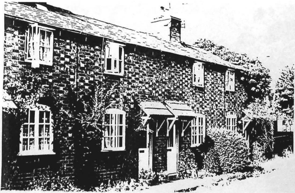
The nineteenth-century brick terrace of four cottages on the north side of Church Lane, the kind of standard row the Victorians added to the village (Conservation Area Study, 1992, fig. 9; 15/08).
