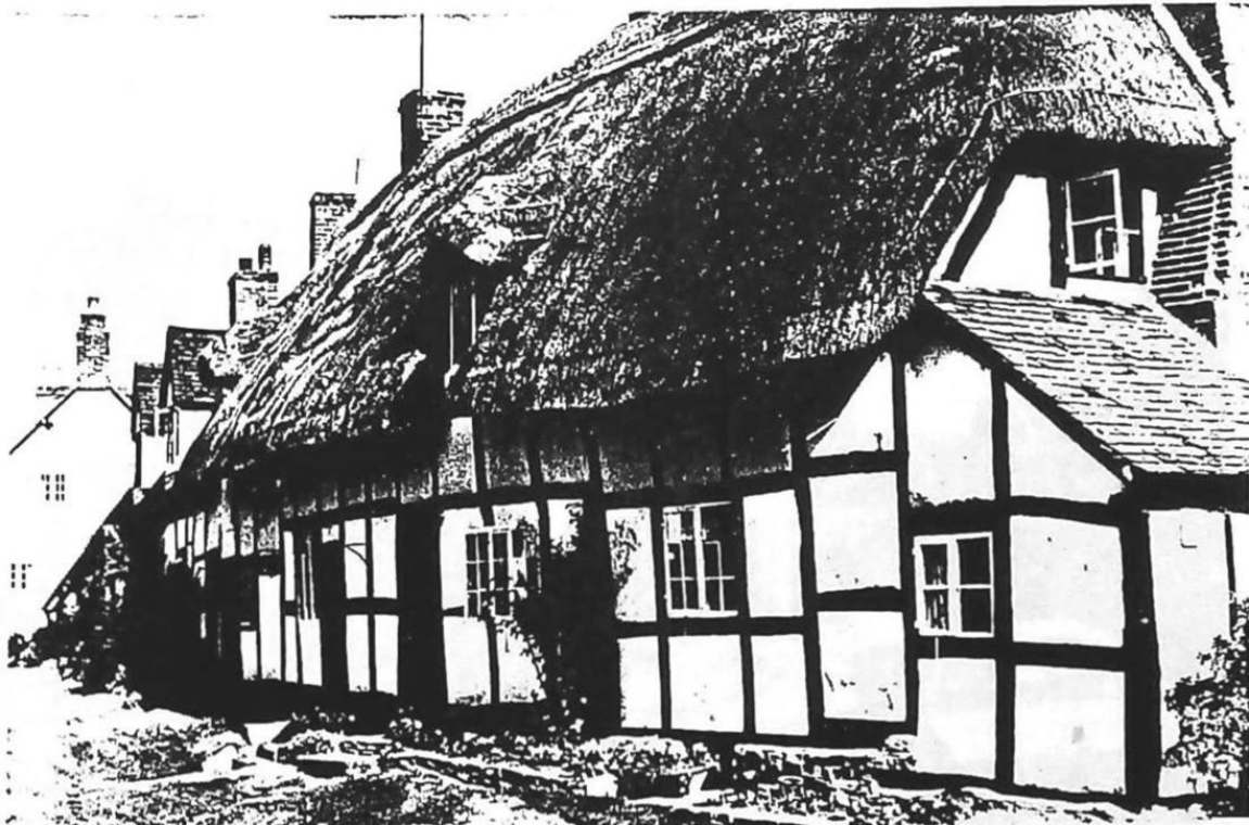
Nos 1–4 Chapel Row, Chapel Street: a seventeenth-century range of four timber-framed cottages under one continuous thatch, "one storey and attic" (Conservation Area Study, July 1992, fig. 54; archive 15/08).
