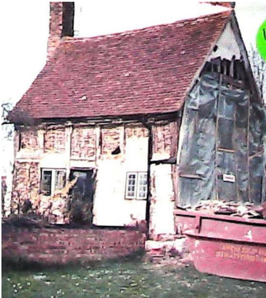
Glebe Cottage, Church Street, at the start of its 1986 restoration. Brick nogging and the remains of wattle and daub show between the oak studs, and a later render patch covers part of the front (16/15).
