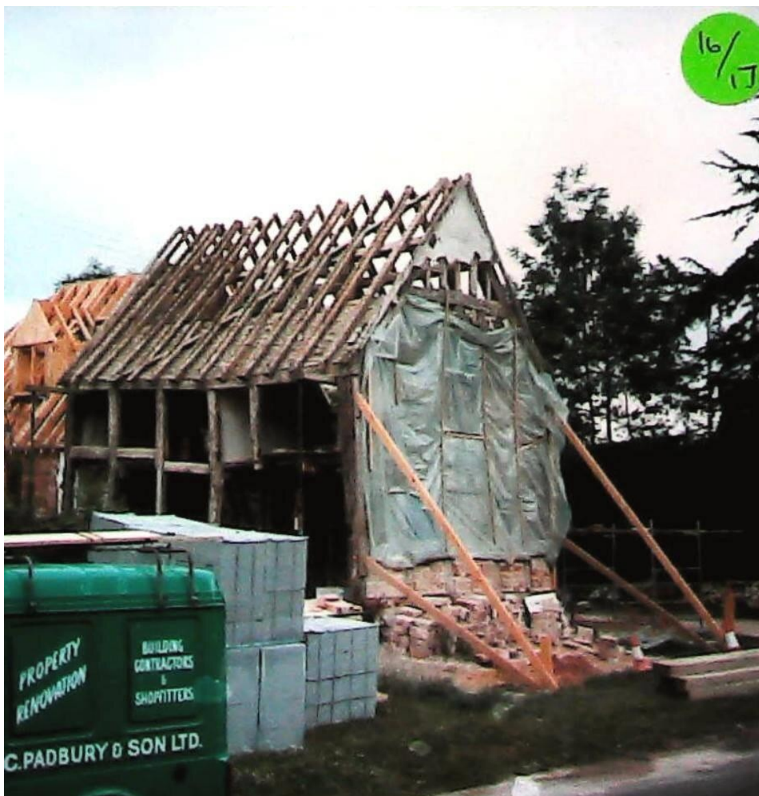
Glebe Cottage stripped to its frame in 1986: bare rafters, open oak studs, a propped gable under plastic, and new concrete blocks stacked by the contractor's van (16/17).
