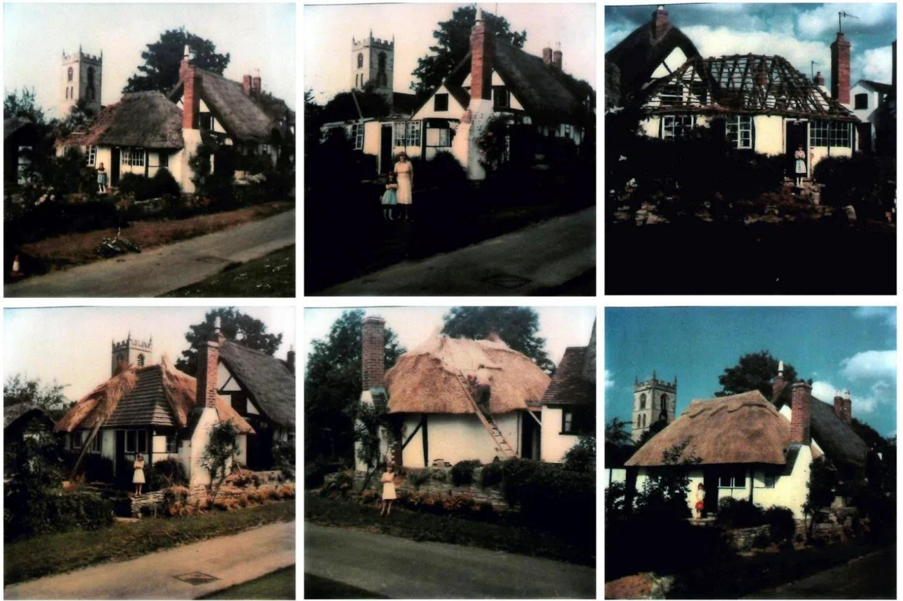
Rethatching "10p Cottage", Boat Lane, August 1980, with St Peter's tower behind: from worn thatch (top left) to stripped rafters and a finished ridge (bottom right) (24/30).
